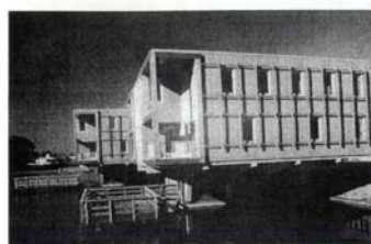
Fig.4 Eastside with platforms
